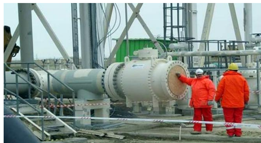
Figure 1-2. The ball valve and point of entry into the 30-inch pipeline
